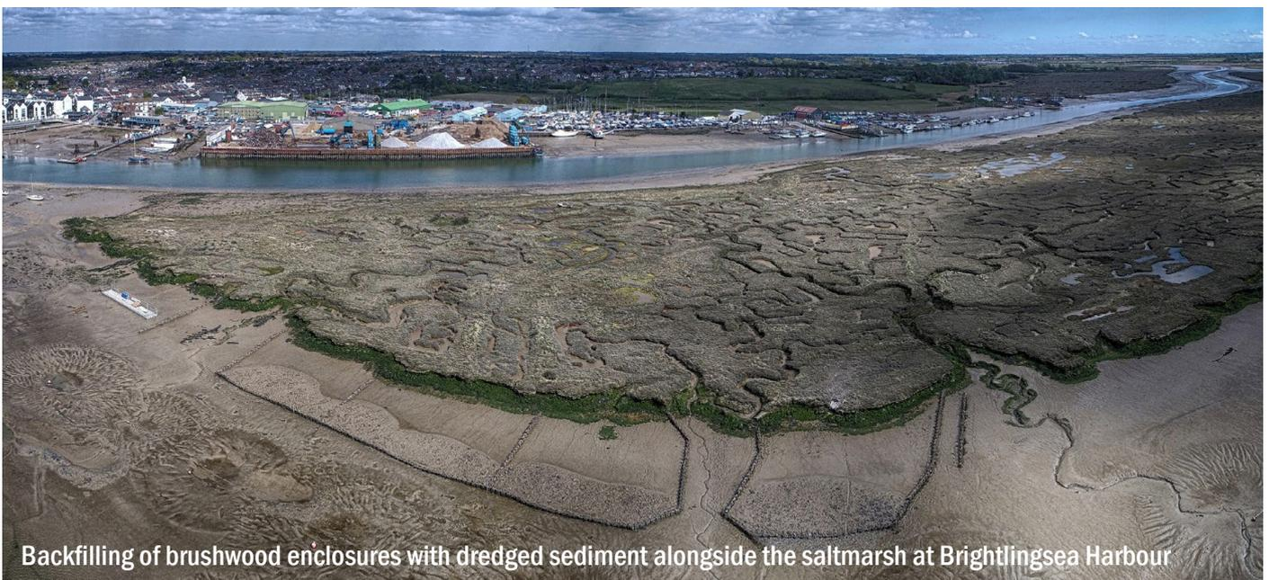
Backfilling of brushwood enclosures with dredged sediment alongside the saltmarsh at Brightlingsea Harbour
