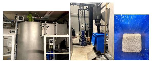
Figure 2. From left to right 2a: struvite reactor, 2b: harvesting system with container, and 2c: struvite produced
