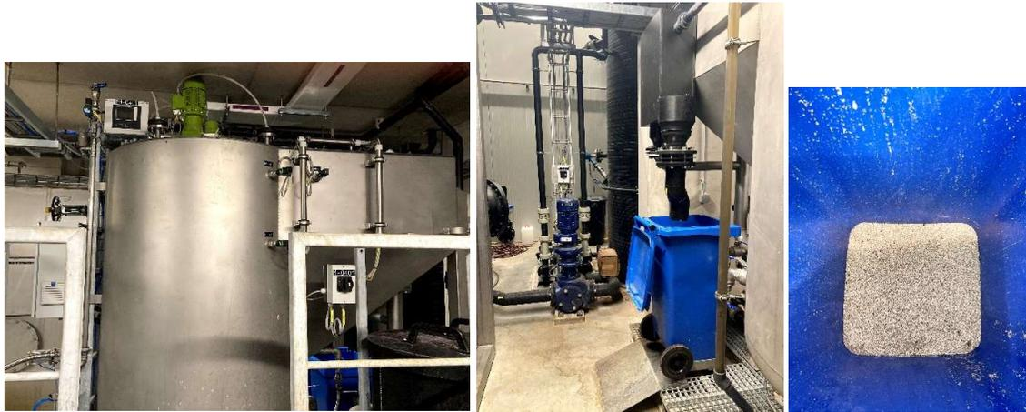
**Figure 2.** From left to right **2a**: struvite reactor, **2b**: harvesting system with container, and **2c**: struvite produced
