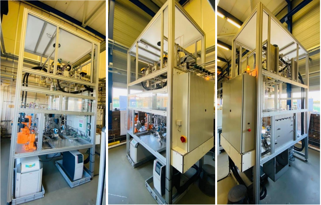
Figure 5: The ATS installation from various sides.
